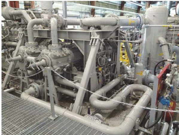
Figure 11: Second PAN Manifold unit installed (with work platforms) – left side view
