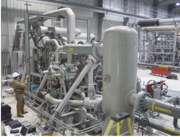
Figure 7: First PAN Manifold unit installed (without work platforms) – left side view
